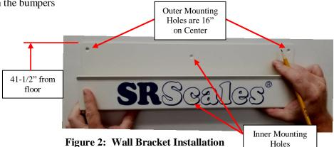
**STEP 5:** For stud walls, use a stud finder and locate any studs in the mounting area:
